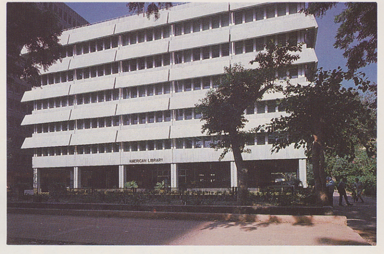
USIS LIBRARY BUILDING AT NEW DELHI
